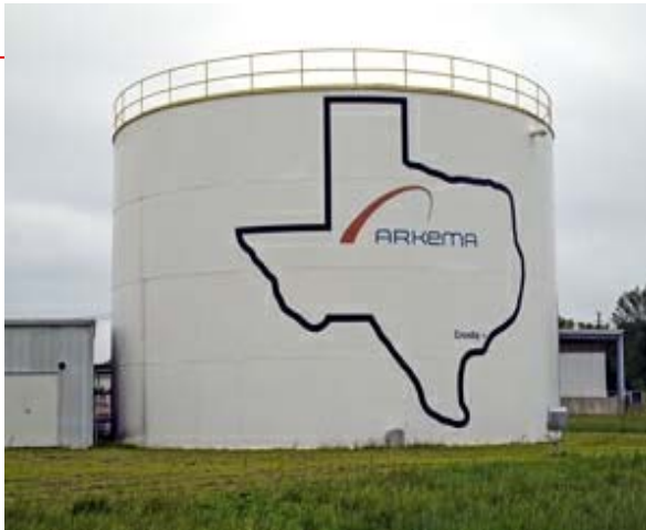
Arkema plant in Crosby, Texas
